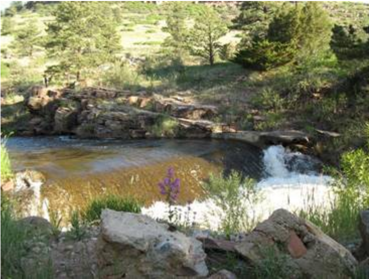
Longmont's South Saint Vrain Creek Diversion Structure
